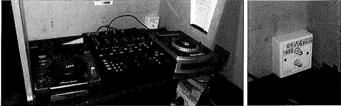
Figure 3: DJ desk controls
